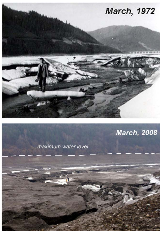
Fig. 13. Ice obstruction of the Bistrita river channel induced a change in the course of the river (Calugareni area in the emersion area of the Izvoru Muntelui Reservoir): March 1972 (photo: I Miron); March 2008 (photo: N. Rădoane).
